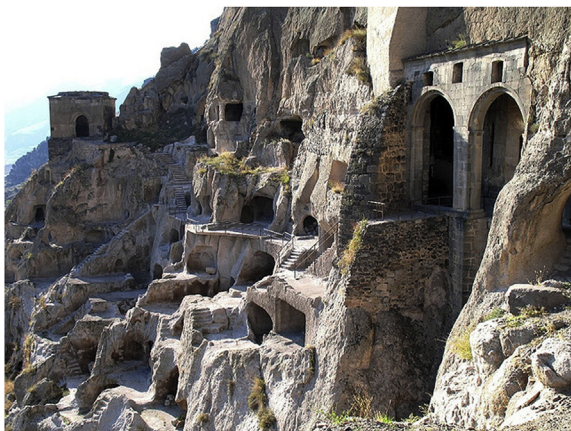
Fig. 1. Front view of Vardzia rock-cut city, which is hewn into Mtkvari ignimbrites flow.
