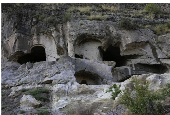
Fig. 12. Part of the Vardzia rock-cut city damaged by the AD 1283 earthquake.
