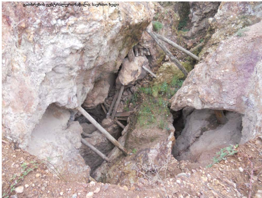
Fig 3 Entrance of the central part of the Kachagiani mine.
