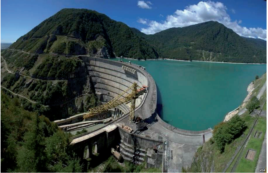
Fig. 37. Dam of the Enguri Power Plant and a part of the water reservoir.
